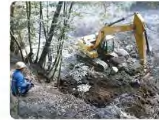
Takachiho No. 3 Emergency Rock Removal (2010)
