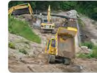
Funaishi River Debris Flow Disaster Recovery (2010)
