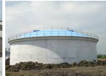
Septic Tank Sludge Treatment
