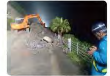
National Route 220 Emergency Recovery (2017)
