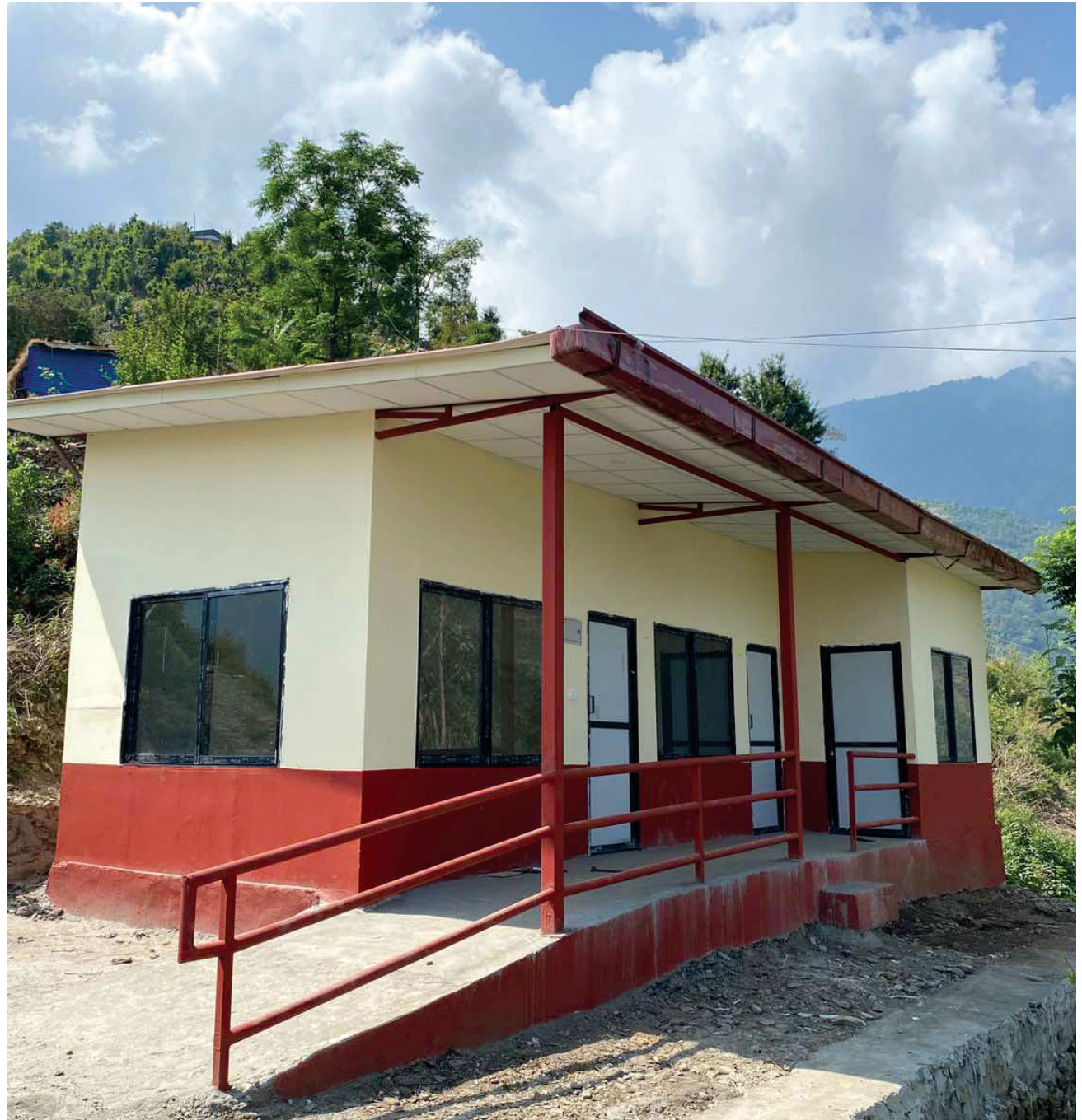
From community consultation to completion: community engagement, technical support, and construction of the prefab building for ward office in Aathbiskot Municipality-12
