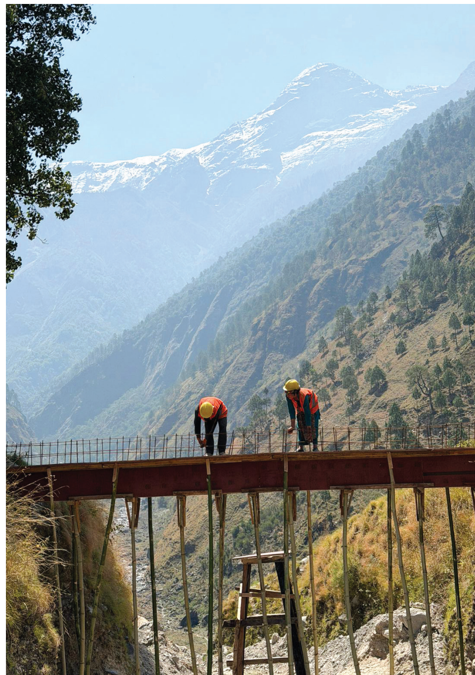
Community participation in the restoration of Holi Pipal Rukh-Benneta irrigation canal in Aathbiskot Municipality-6
