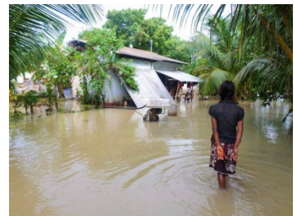
Flood damage to the infrastructure in the dry zone of Sri Lanka 2015. Source: Red Cross Sri Lanka
