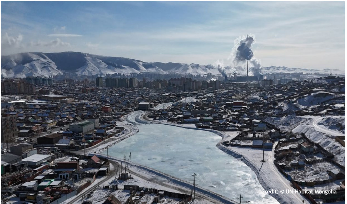
Photo 3. Flood protection channel and retention basin capturing water and ice in the Tolgoit River basin during the 2025-2026 winter
