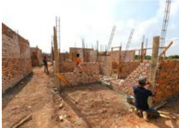
House under construction (Indonesia)
