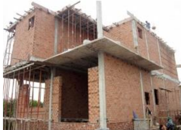
House under construction (Vietnam)
