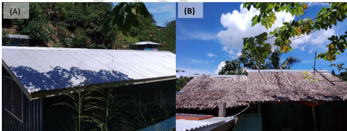
Figure 56. Examples of metal (A) and traditional materials (B) roof.
