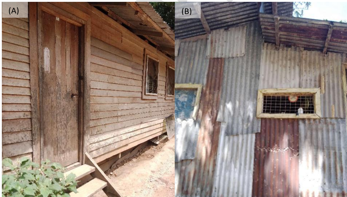
Figure 58. Examples of wood (A) and metal (B) walls.
