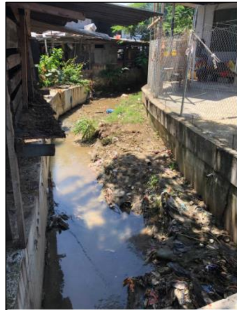
Figure 11: Stormwater drain through Ontong Java (Credit: Usha Iyer-Raniga)
