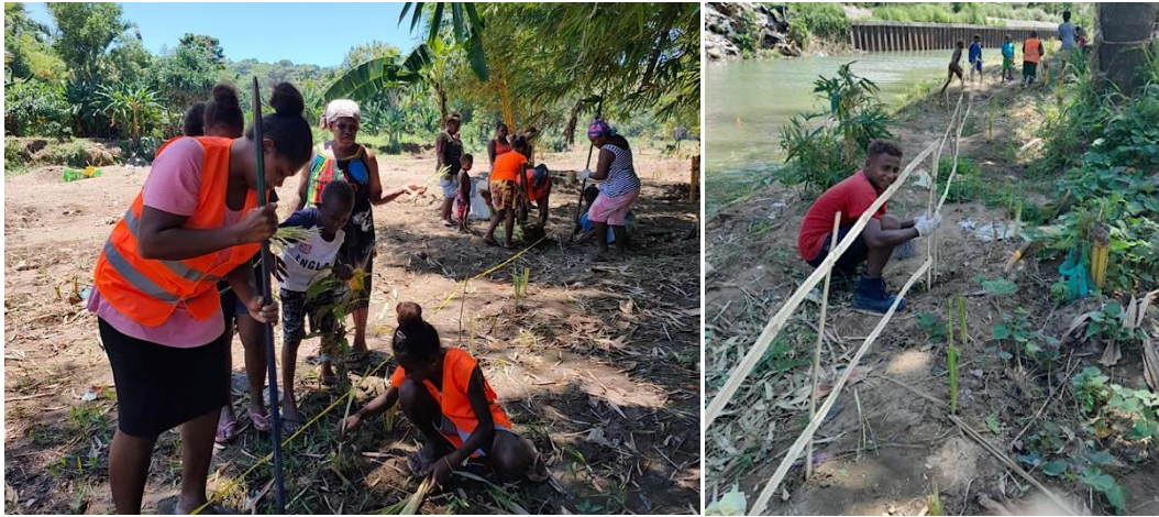
Vetiver grass planting, bamboo replanting and fencing installation on riverbank
