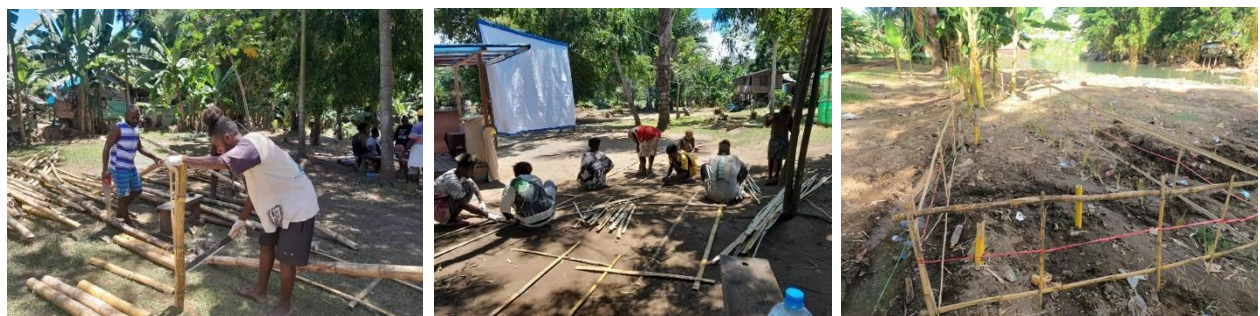
Bamboo fencing constructed to help protect vetiver grass and young bamboo along riverbanks
