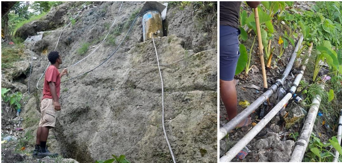
Central Valley landslide risk hotspot in Zone 27 with community-built water pipes
