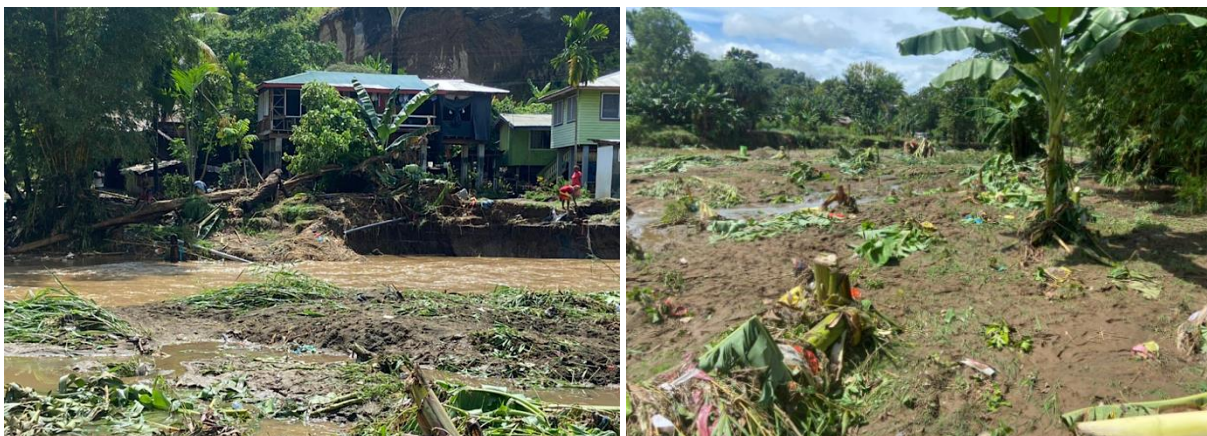
Flooding debris and damage along Mataniko riverbank (zone 27)
