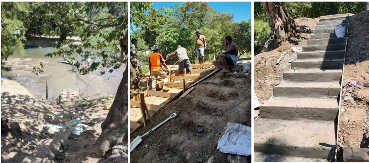
Steps and jetty before construction (left). Stairway construction (middle and right)
