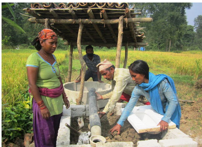
Community enthusiasm to build toilets
