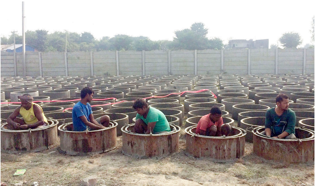
Local masons widely engaged in producing concret rings for toilet construction
