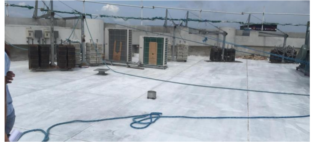
Building roof with high SRI paint
