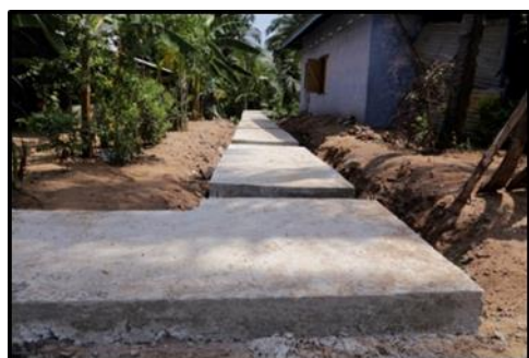
The completed drain with concrete slabs for reinforcement
