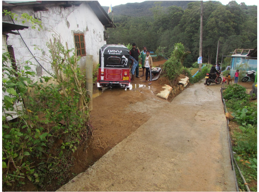
The completed internal access road in Kikiliyamana GN division.
