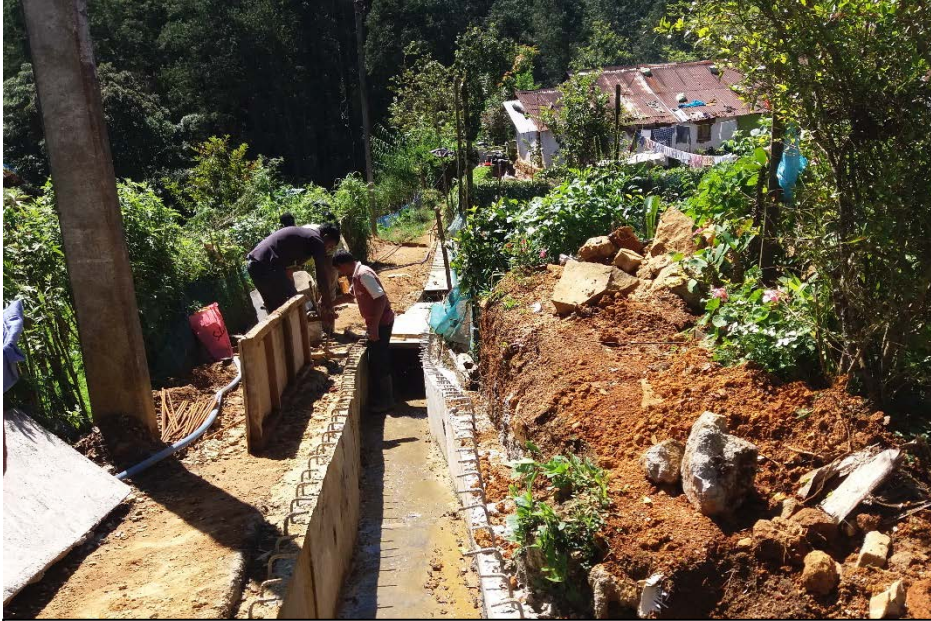
The internal road during construction.
