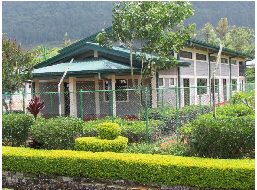
The MPCC at Medakumubura estate is nearing completion.
