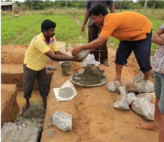
Foundation work in progress.
