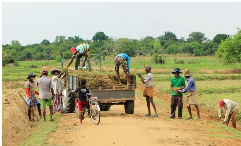
Turfing of the road side in progress.
