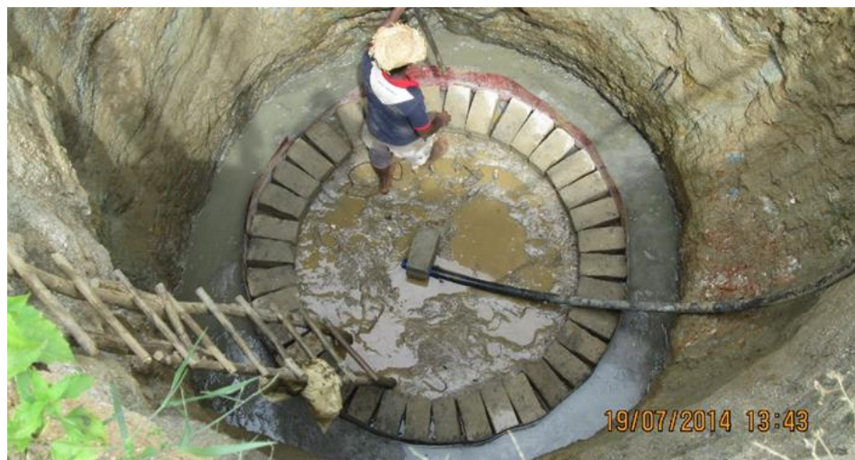
Construction of the new well in progress.
