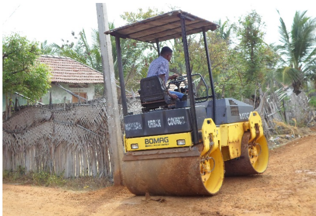
Repair work in progress along the 50 Housing Scheme Road
