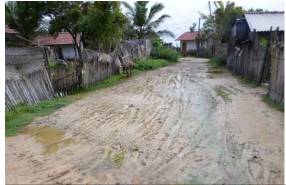
50 Housing Scheme Road before rehabilitation
