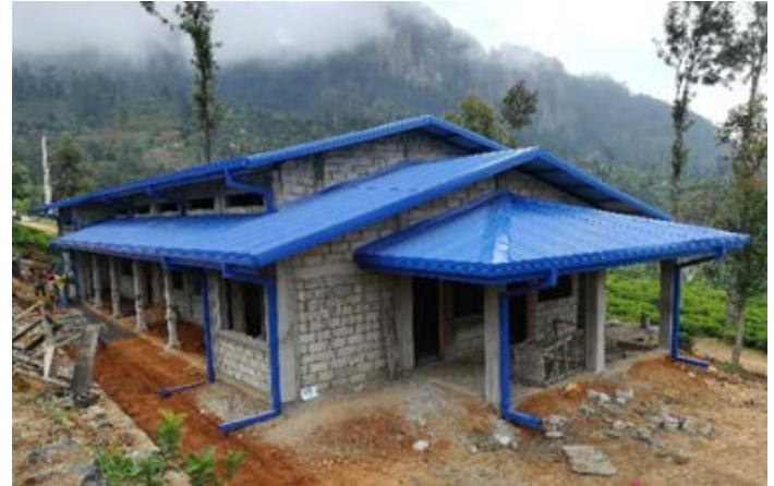
The MPCC is nearing completion at Liddesdale estate.
