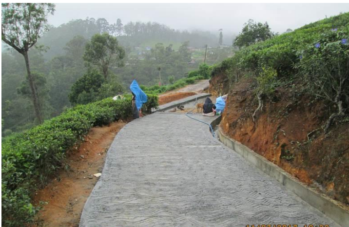
The completed stretch of the road with storm water drain.
