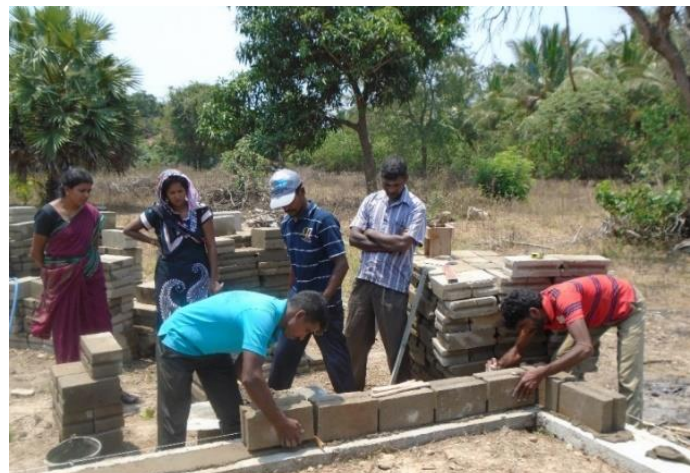
Construction training of the super structure in progress.
