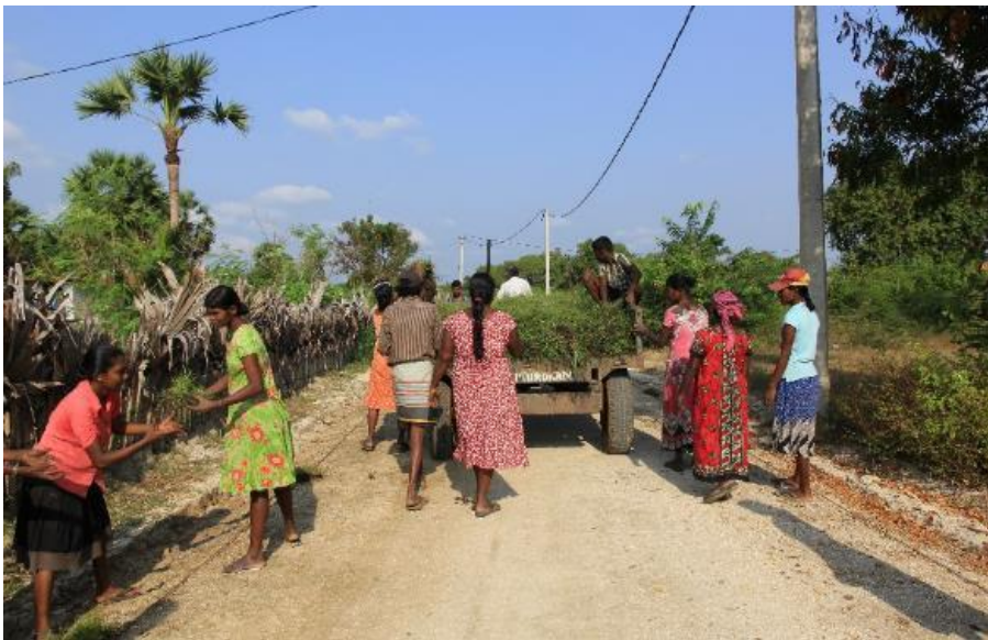
Turfing of the roadsides in progress by the WRDS members,
