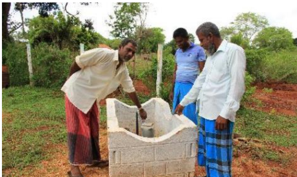
Palaikuli RDS members inspecting the tube well
