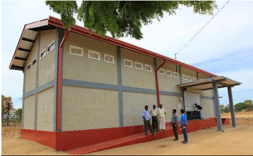
The Periyaparathan community storage facility
