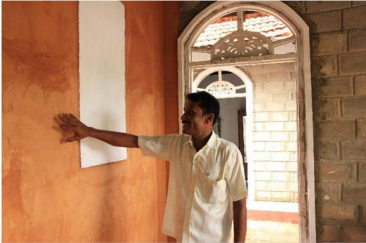
The completed house has interior walls constructed with fair faced cement blocks and mud plastering. The courtyard is in the background.
