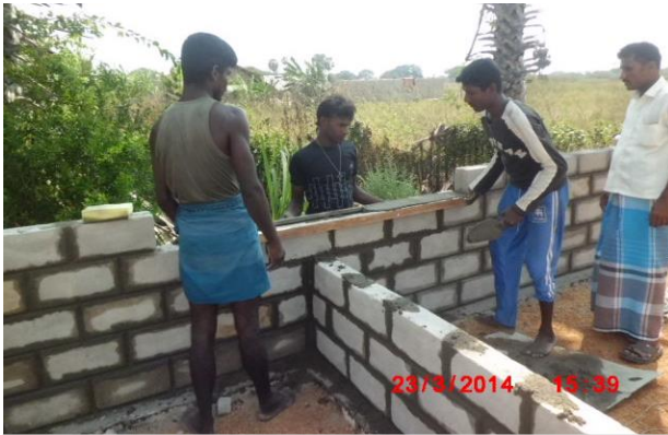
House construction in progress using fair-faced cement blocks
