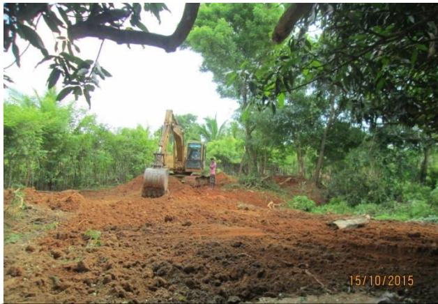
Road during construction.
