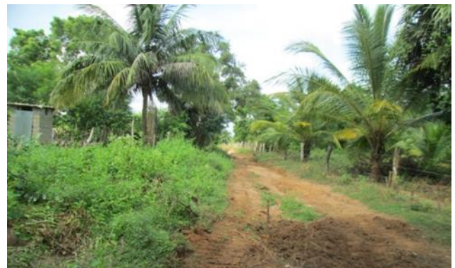
Internal road before rehabilitation.
