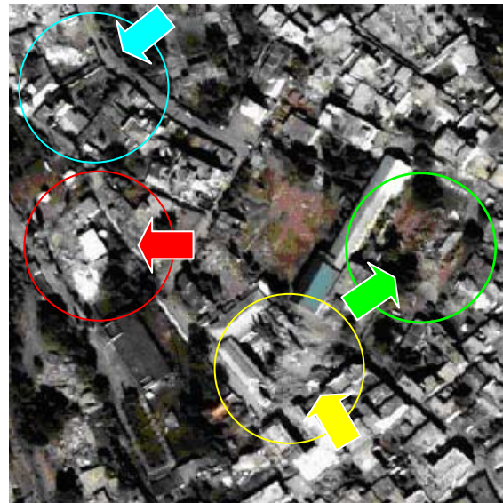
Infrastructure Damaged After the Earthquake
