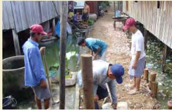
During upgrading process.
