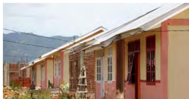
Housing constructed through a process led by the tsunami survivors themselves.
