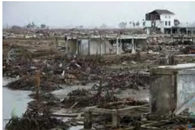
Total devastation in Banda Aceh caused by December 2004 tsunami.
