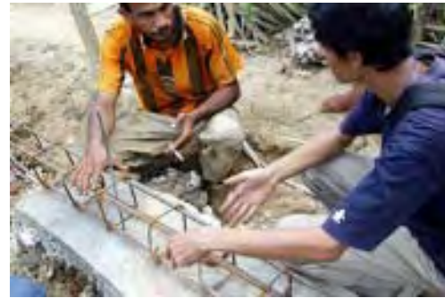
A tsunami survivor manages his house construction.
