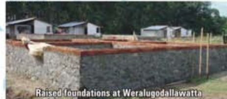
Raised foundations at Weralugodallawatta
