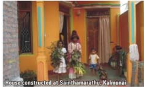
House constructed at Sainthamarathu, Kalmunai
